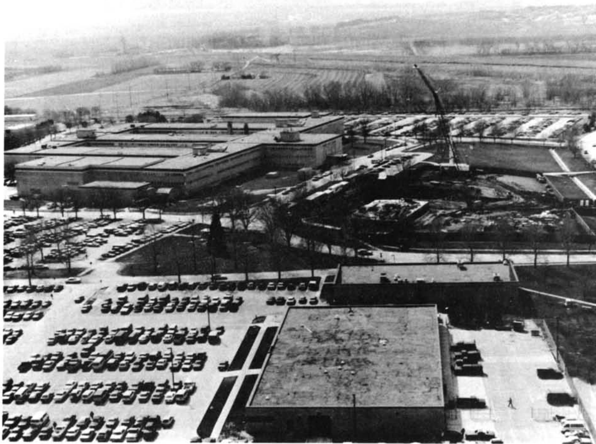
SAC COMMAND CENTER UNDER CONSTRUCTION, 1988
